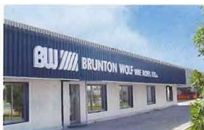
View of the Plant office
